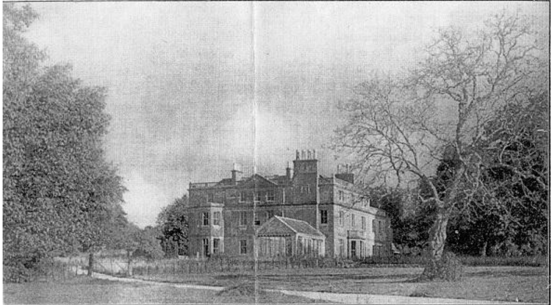
Cowesfield House, Whiteparish, the 20-room mansion which was formerly the home of the late Mr. W. F. Lawrence, once Postmaster-General, and which is to be demolished. Unoccupied since the war, its boundaries are still skirted by rolls of barbed wire as a reminder of Allied military requisition. First stages of demolition will be on Wednesday when everything within the walls is to be dismantled. Six thousand square feet of flooring and 100 doors are among the listed items. When these have been removed demolition contractors will begin work on the mansion's skeleton.
